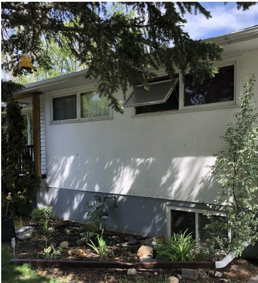
Before (window enlargement & painting)
